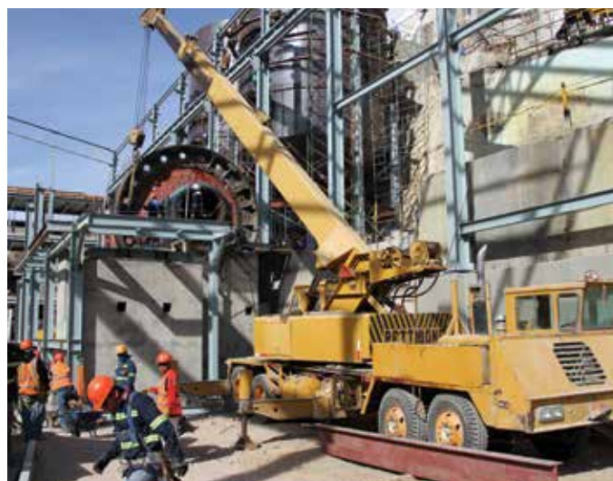
Installing the new ball mill at El Cubo
